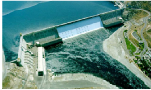
Large Scale SCADA Systems
